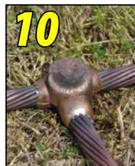
10 Remove weld and clean mold before making next connection.
