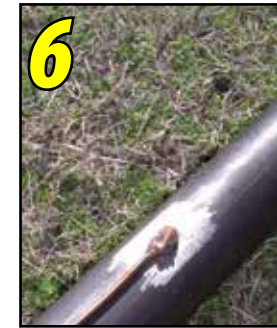
6 Remove and clean mold before making next connection.
