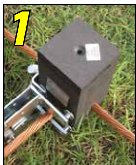
1 Position cleaned conductors in mold.
