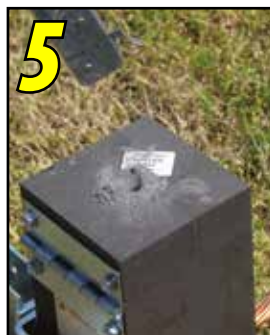
5 Ignite the starting powder with the Flint Ignitor.
