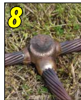
8 Remove weld and clean mold before making next connection.
