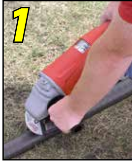
1 Clean pipe before making weld.
