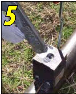
5 Close lid and place starting powder on top. Ignite starting powder with Flint Ignitor.
