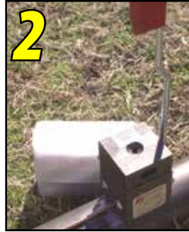
2 Position conductor and mold onto pipe.
