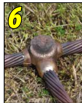
6 Remove weld and clean mold before making next connection.
